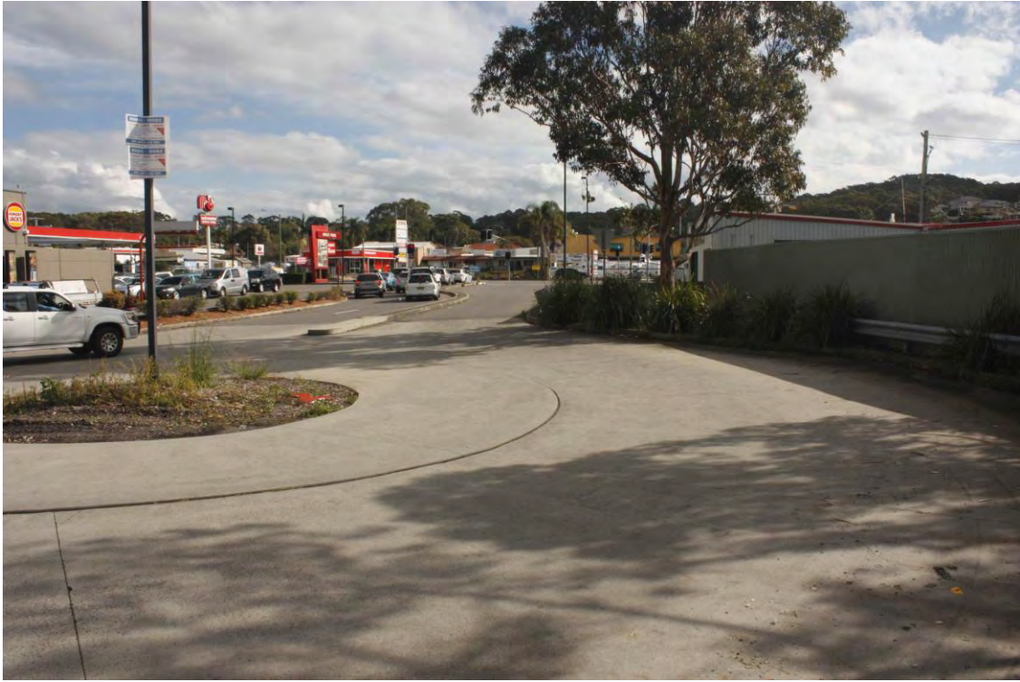
Photo No. 3: Looking generally west towards the Pacific Highway showing the existing service road to the existing retail / hospitality complex and signalized intersection.
